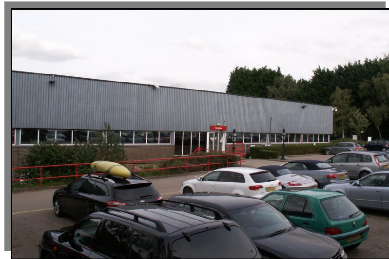
Extensive Car Parking
